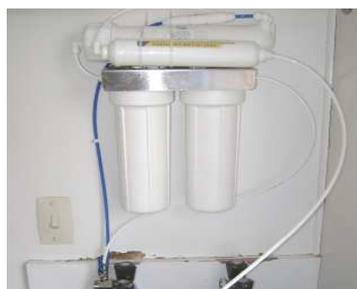
Portable RO set up in a laundry.
